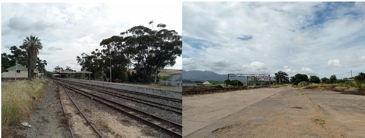
Figure 4-4: Current conditions of the infrastructure Botriver rail station
